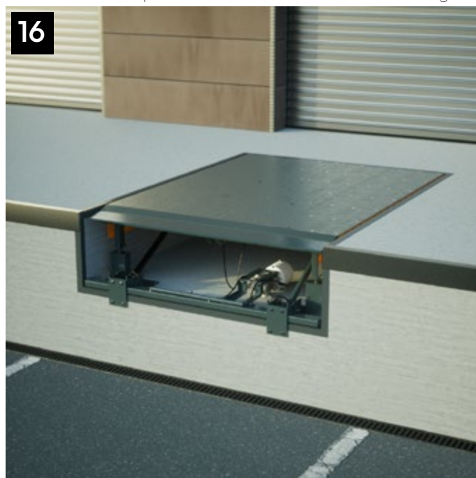
Rampa correttamente installata / Ramp correctly installed.
