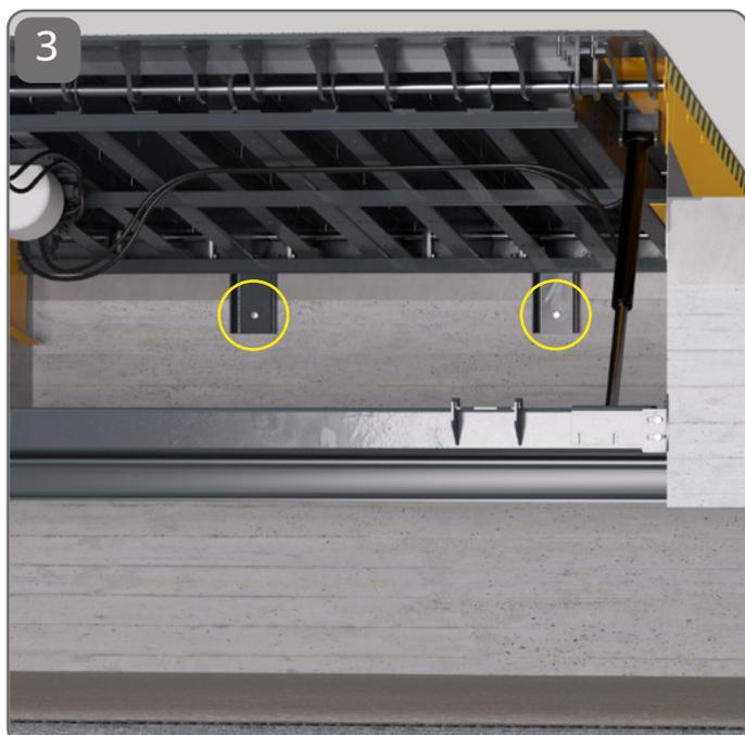
Fissare a muro la cerniera posteriore mediante tassellatura di adeguata dimensione / Secure the rear hinge to the wall by screwing with the appropriate-sized anchor
